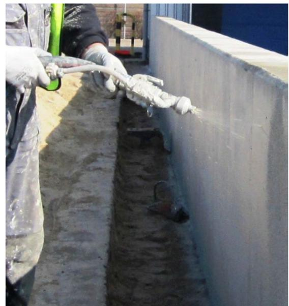
**Image 2: Spray application of MasterSeal 6100 FX**
