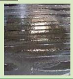
As torching continues, the heat-adhesive strips will assume a semi-liquid, glossy consistency: the surface is now ready to receive the panels or rolls of insulation.
