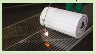
The THERMOBASE rolls which are unrolled on the surface just torched must be bonded to the TECTENE BV STRIP EP by pressure over the whole surface of the roll, exerted by the operator simply treading on them (this must be done over the entire surface of the panel or roll).
