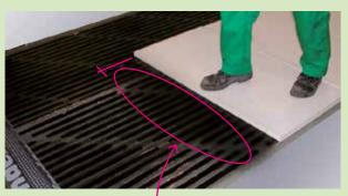
The insulation panels laid on the surface just torched must be bonded to the TECTENE BV STRIP EP by the pressure of the operator simply treading on them (this must be done over the entire surface of the panel).
