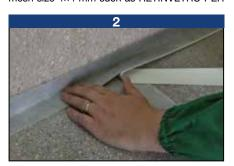
RASANTI onto the first coat of **GEOFLEX**.
