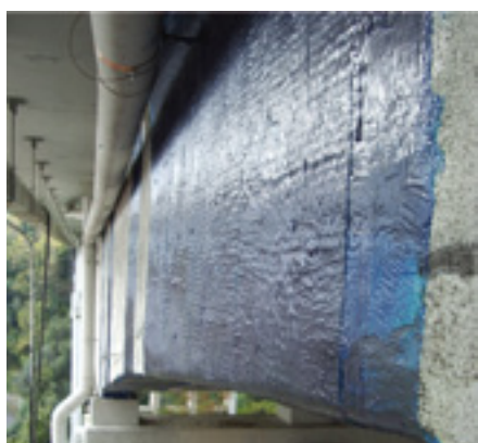
6.2.1 MasterBrace U strapping to reinforce against shear
