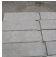
6.1.7 Sandblasting is essential in plating interventions
