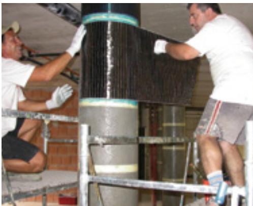
6.3.1 Confinement of a reinforced concrete column
